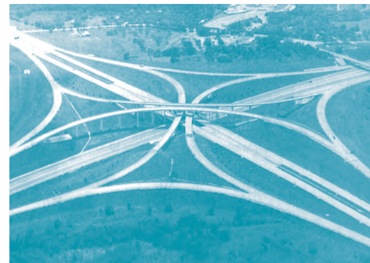
Example of a four level interchange
