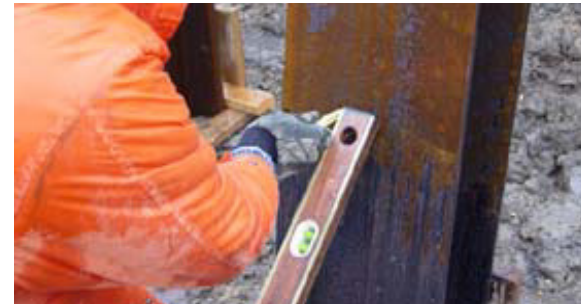
Figure 10 Continue Driving Until Bearing
