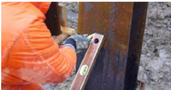
Figure 7 Mark pile as Driving Continues
