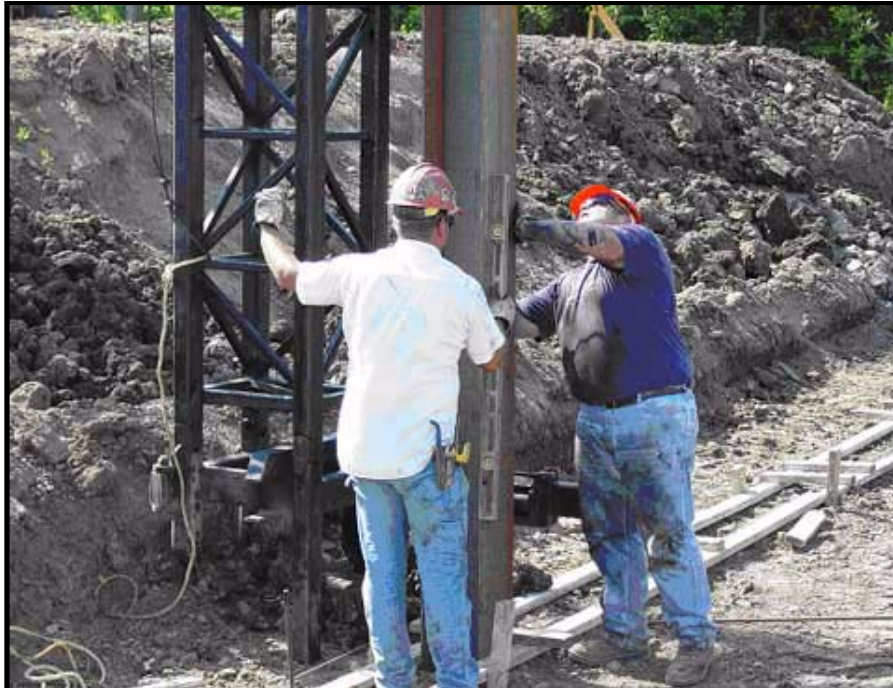
Figure 5 Plumbing an H-Pile
