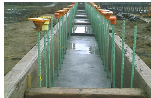
Figure 8 Embedded Epoxy Reinforcement
