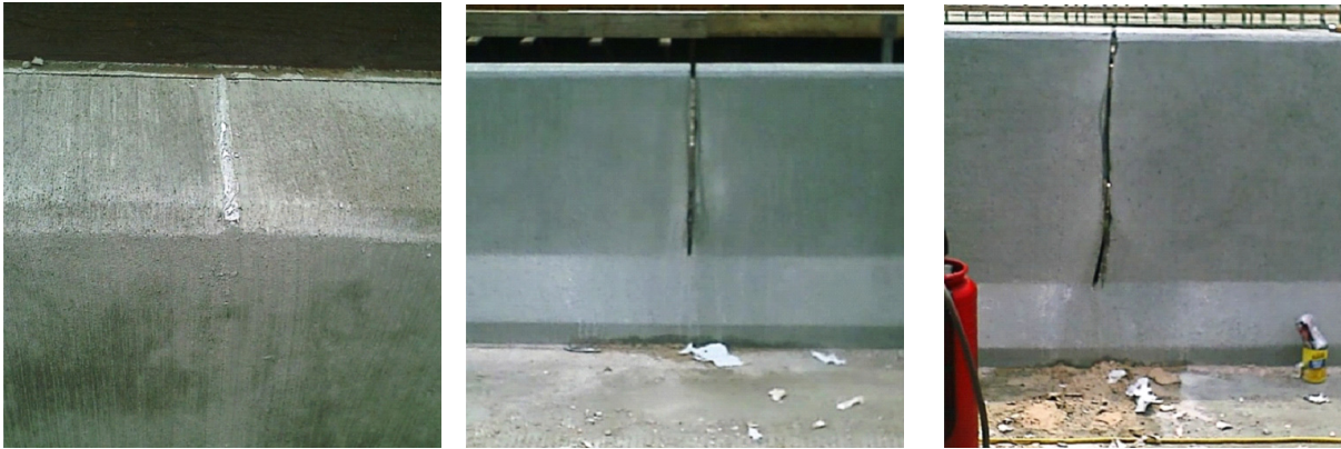
Expansion Joints: Before Removal, After Removal (Good), After Removal (Bad)
