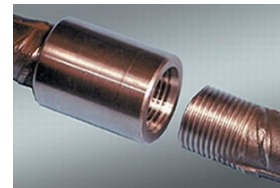
Figure 4: Threaded Splice
