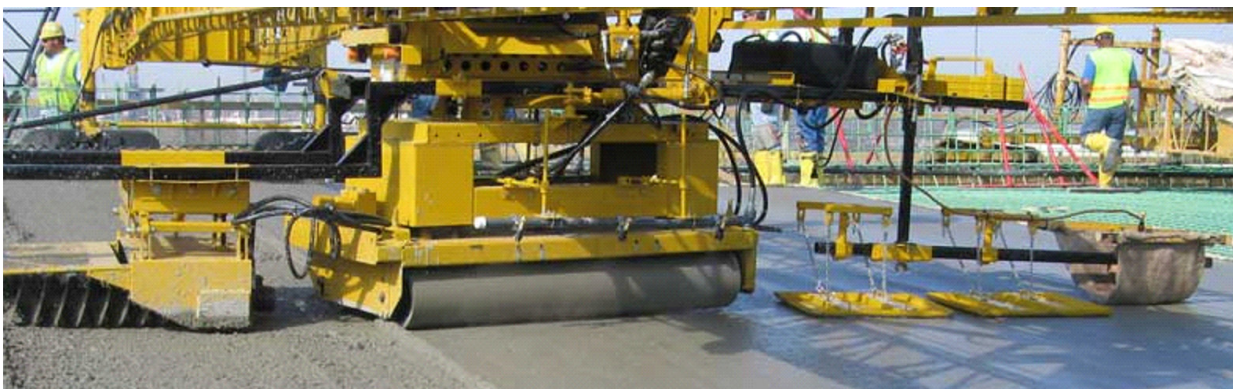
Figure 11 Deck Finishing Machine
