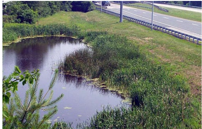
Figure 3.8 Wet Detention Basin
