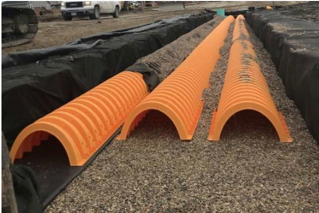
Figure B.3 Open Bottom Underground Storage
