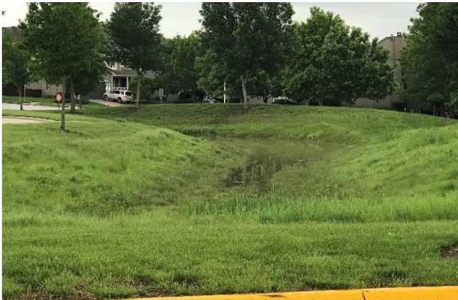
Figure 3.7 Dry Detention Basin
