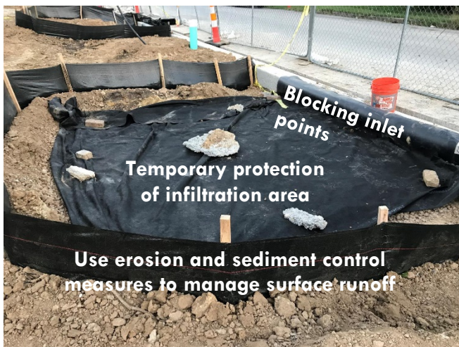
Figure 4.10 SCM Protection Measures
