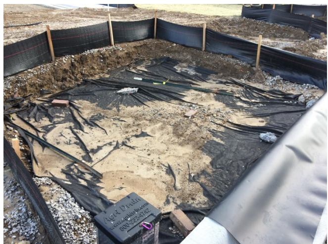
Figure 4.11 Protected SCM After Rain Event
