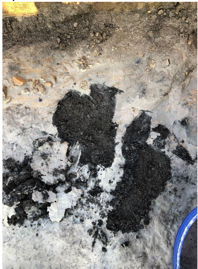
Figure 4.7 Growing Media Revealed Underneath Layer of Fines
