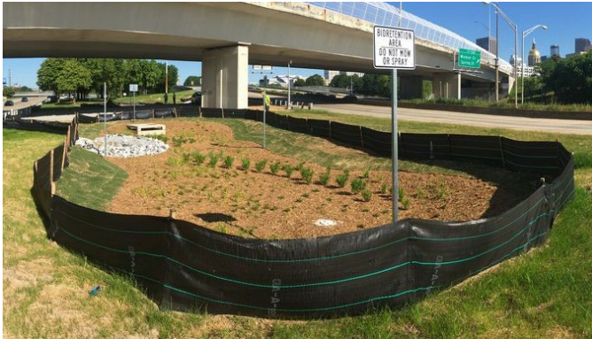
Figure 3.5 Newly Constructed Bioretention Basin
