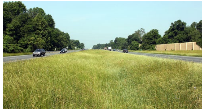
Figure 3.2 Stormwater Right-of-Way (Median)
