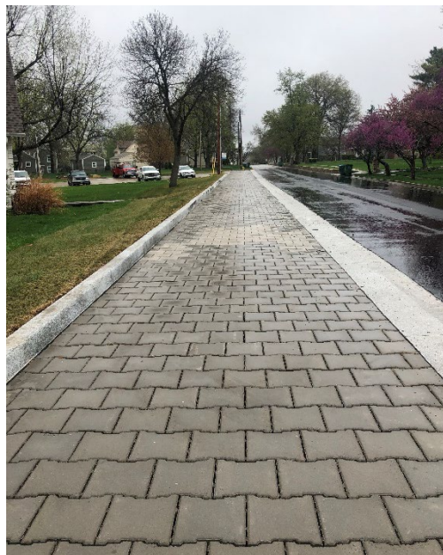
Figure B.1 Permeable Paver Shoulder
