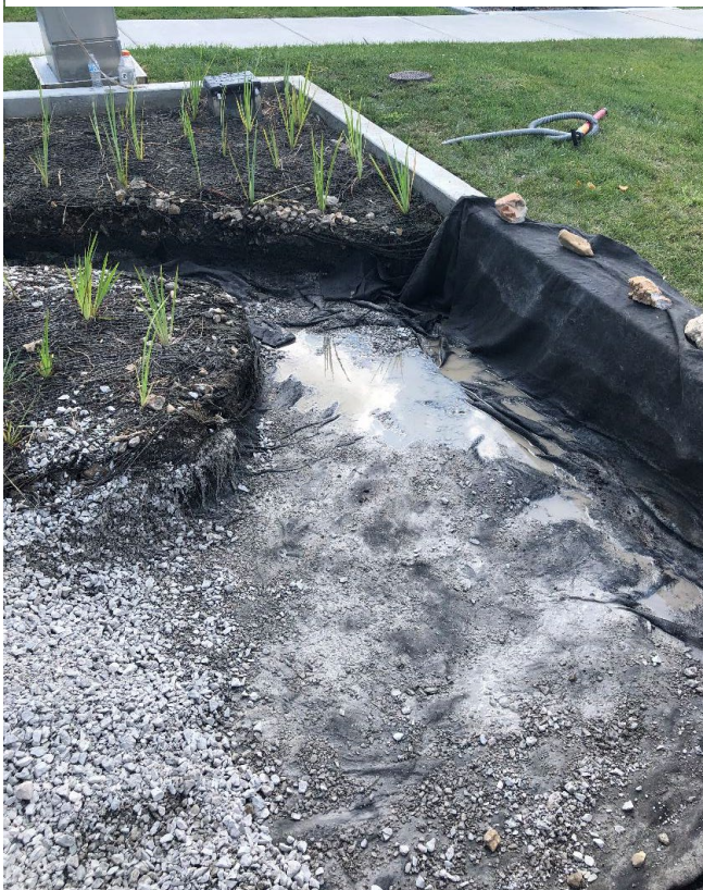
Figure 4.6 Layer of Fines Preventing Infiltration
