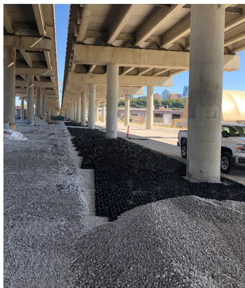
Figure B.2 Grid Pavers
