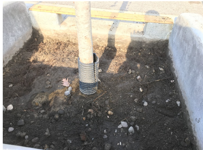
Figure 4.9 After – SCM Was Excavated to Provide Designed Ponding Depth
