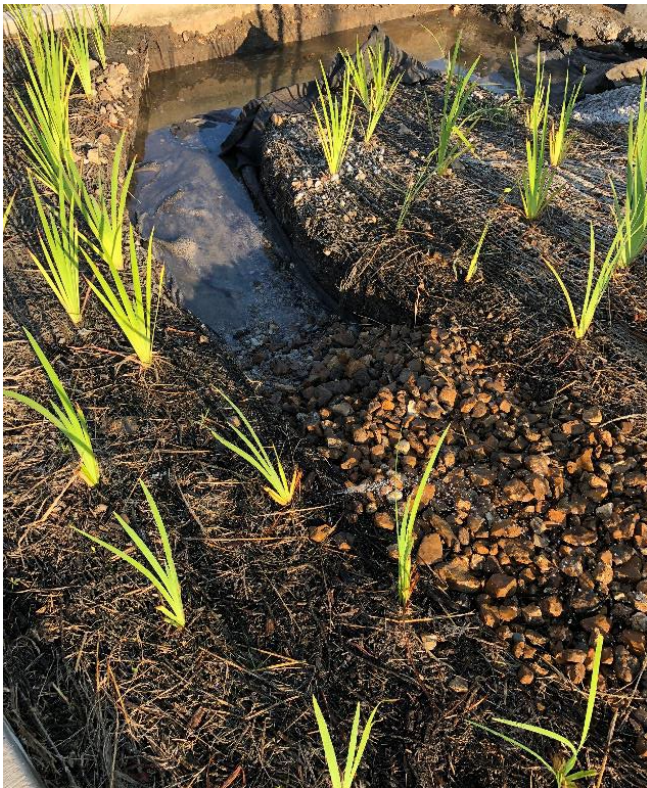
Figure 4.6 Layer of Fines Preventing Infiltration
