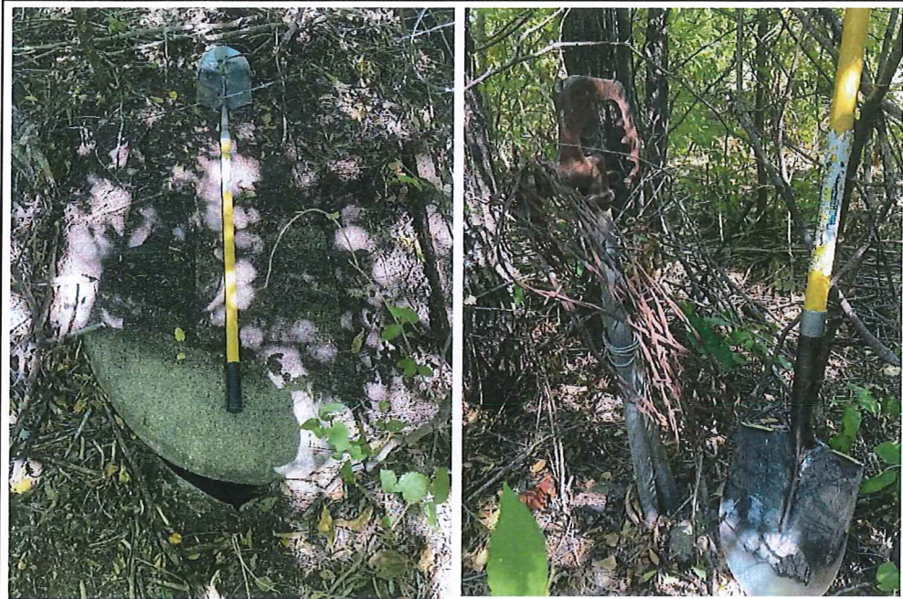
Figure 4.5. Two images showing a concrete, oval-shaped sewer (left), and a hand pump (right). Shovel is shown for scale.
