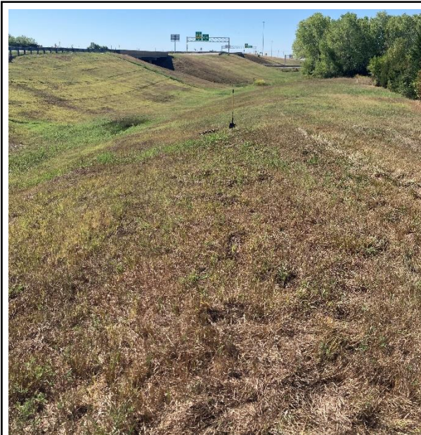
Figure 4.1. Image showing disturbances on the west side of K-96, facing south.
