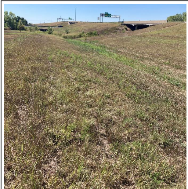
Figure 4.2. Image showing disturbances on the east side of K-96, facing south.
