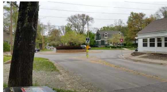
Looking east to Barker Roundabout.
